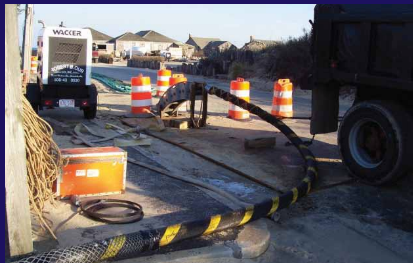
Once the submarine cable is laid, it is then connected to an underground cable inside a manhole near the shore.
